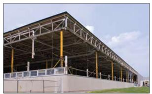
With jacks in place, support pillars and walls are cut. The roof is inched up to its new position.
